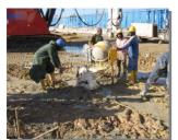
Post test grouting of a working pile
